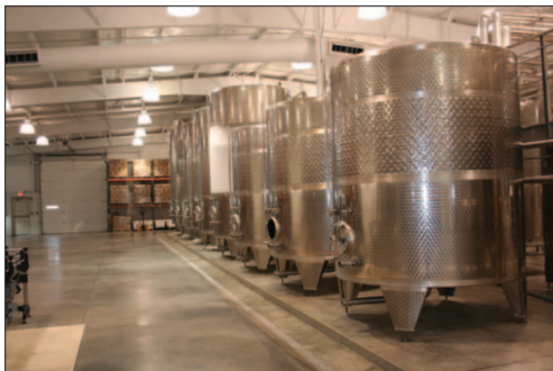
Figure 4. Modern wineries ferment in stainless steel tanks that are jacketed so that glycol circulation can be used to control temperature. (Photo courtesy of Prospero Equipment Corp.)
