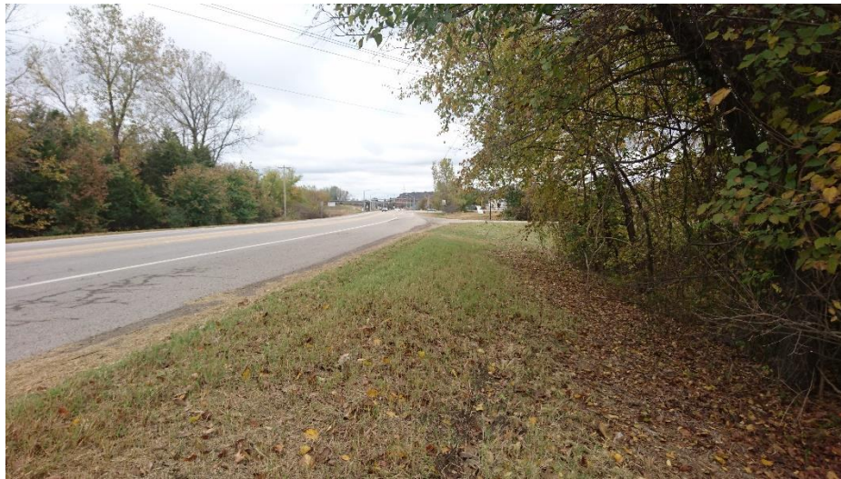
Figure AII.3 – Current situation of proposed location of CAM#4,, in Zone B
