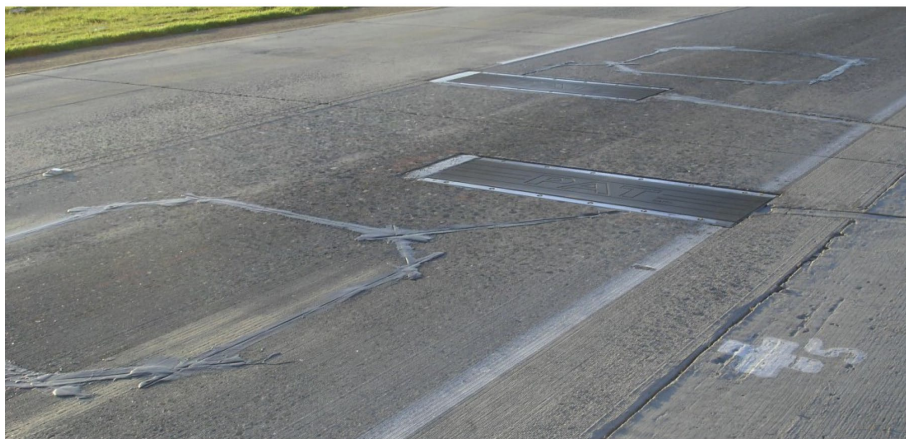
(a) Bending Plate Weight Sensors in a Staggered Configuration (Type I)
