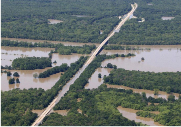
(A) Flooding Closes I-40 in Arkansas in May 2011 (Ref: CNN.com)
