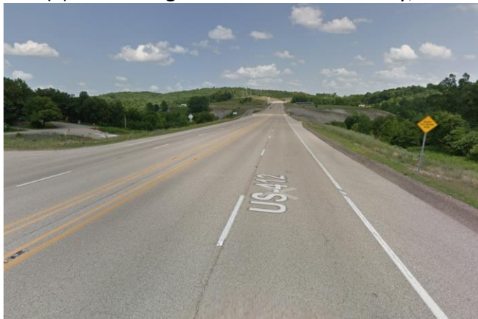
(b) View along the Bypass in Hardy, AR
